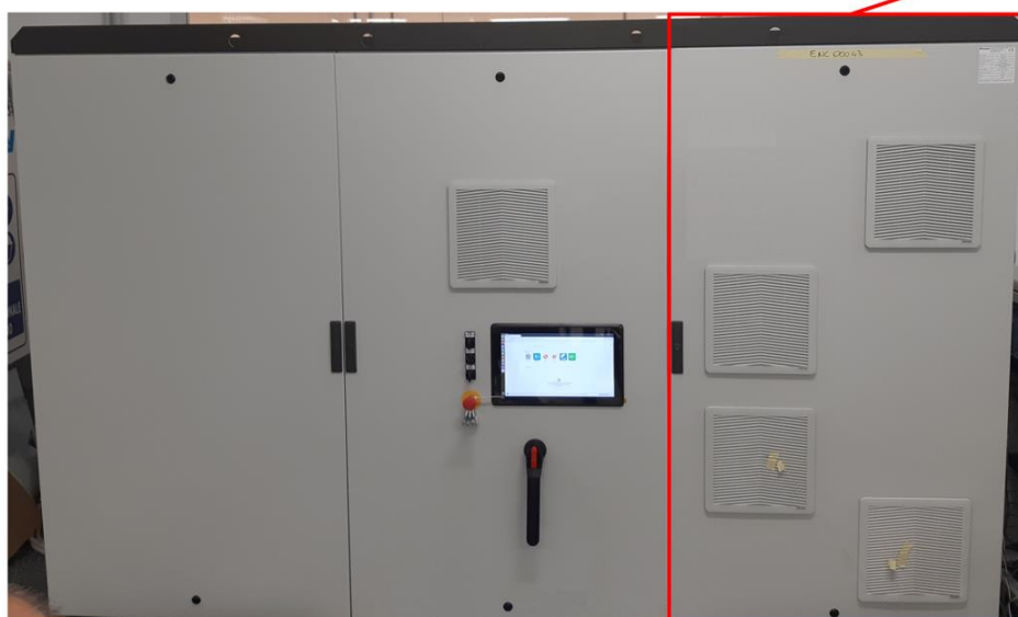
Figure 9 DWSC Electrical Panel, LH Section
