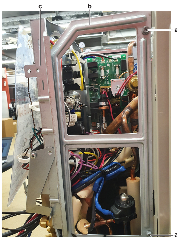
a Screw b Switch box supporting plate c Switch box
