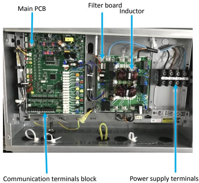
Figure 5-1.2: 8-12HP bottom layer of electric control box
